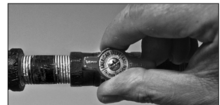
Figure 48: Gas valve in “on” position.
