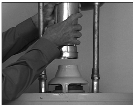
Figure 14: Disconnect the vent pipe (roof jack) from the draft hood.
