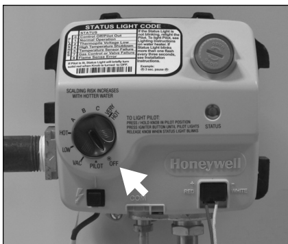
Figure 43: Gas control/valve.
