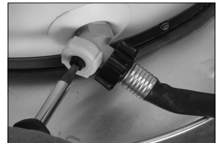
Figure 12: Draining the old water heater.
