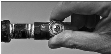
Figure 30: Gas valve in "on" position
