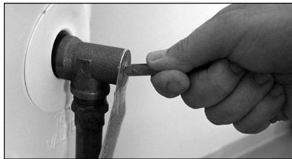
Figure 41: T&P Relief Valve.
