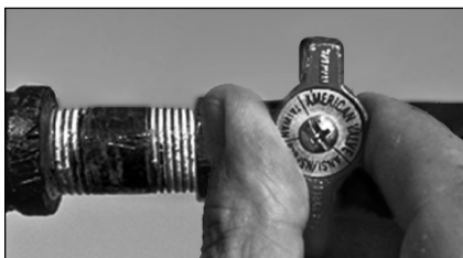
Figure 44: Gas valve in “off” position.
