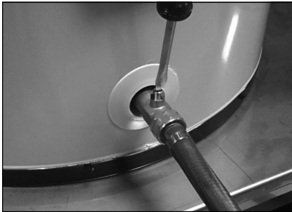
Draining the old water heater.
