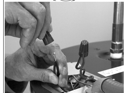
Connecting the electrical wires.
