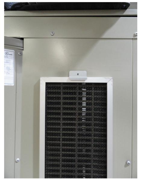
**Figure 6. Top Air Filter Bracket**
