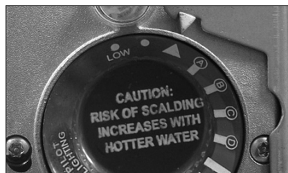
Figure 37 - Adjust the gas control knob to "▲".
