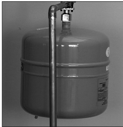
Figure 29 - The Thermal Expansion Tank should be pressurized with air, using a hand pump, to match the home's incoming water pressure.
