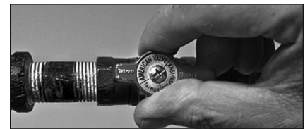
Figure 50 - Gas valve in "on" position.
