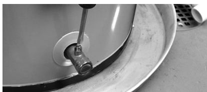
Figure 40 - Draining the water heater.
