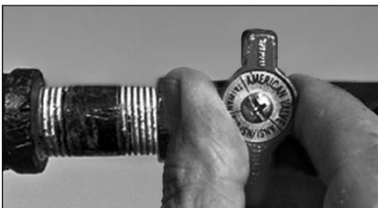
Figure 46 - Gas valve in "off" position.
