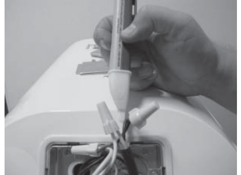
Figure 28 - Non-Contact Circuit Tester
