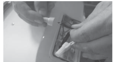
Figure 18 - Connecting the electrical wires.
