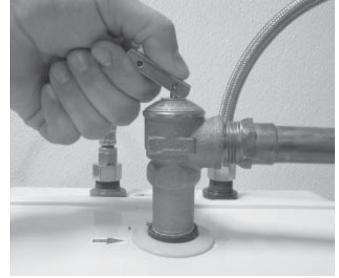
Figure 31 - T&P Relief Valve
