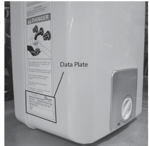
Figure 17 - The water heater’s electrical requirements can be determined from the data plate.
