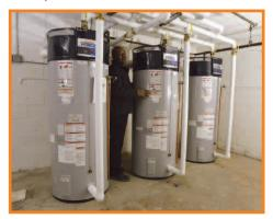
addressed. "Many commercial water heaters require a chimney or stack, and we didn't have that option on this job," said Sparrow. It was necessary to install water heaters with a direct vent/power vent option. The Ultra Force models were installed with vent runs ranging from 6 to 10 feet, which eliminated concerns about indoor ventilation and air quality by venting through a nearby wall.
