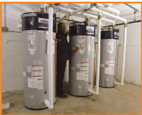
addressed. "Many commercial water heaters require a chimney or stack, and we didn't have that option on this job," said Sparrow. It was necessary to install water heaters with a direct vent/power vent option. The Ultra Force models were installed with vent runs ranging from 6 to 10 feet, which eliminated concerns
