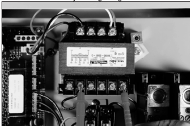
Figure 33. 120 VAC Control Circuit Winding Voltage Tests
