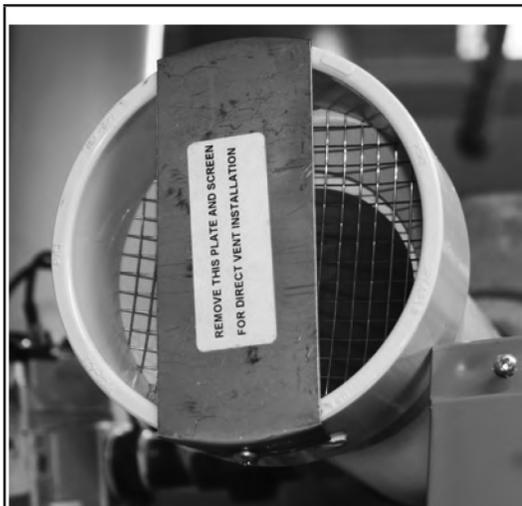
Remove the balance plate (SUF 400/500 only) and air intake screen before gluing intake air pipe to the fitting.
